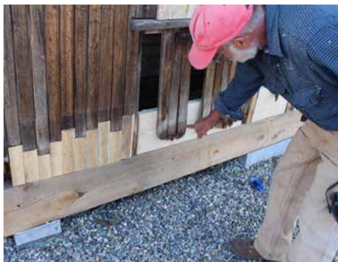
General contractor Mike Perschbacher demonstrates how missing and damaged sections of historic siding on the Como Depot are being careful restored to match their historic appearance.
